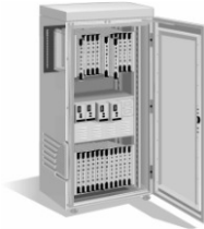
Telecommunications System Indoor Cabinets 户内通讯机柜
